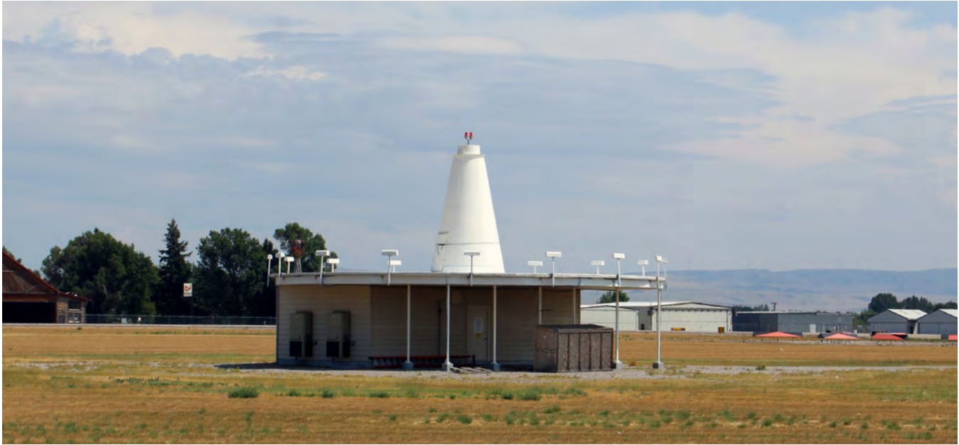
Figure 4.29: Very High Frequency Omnidirectional Range
