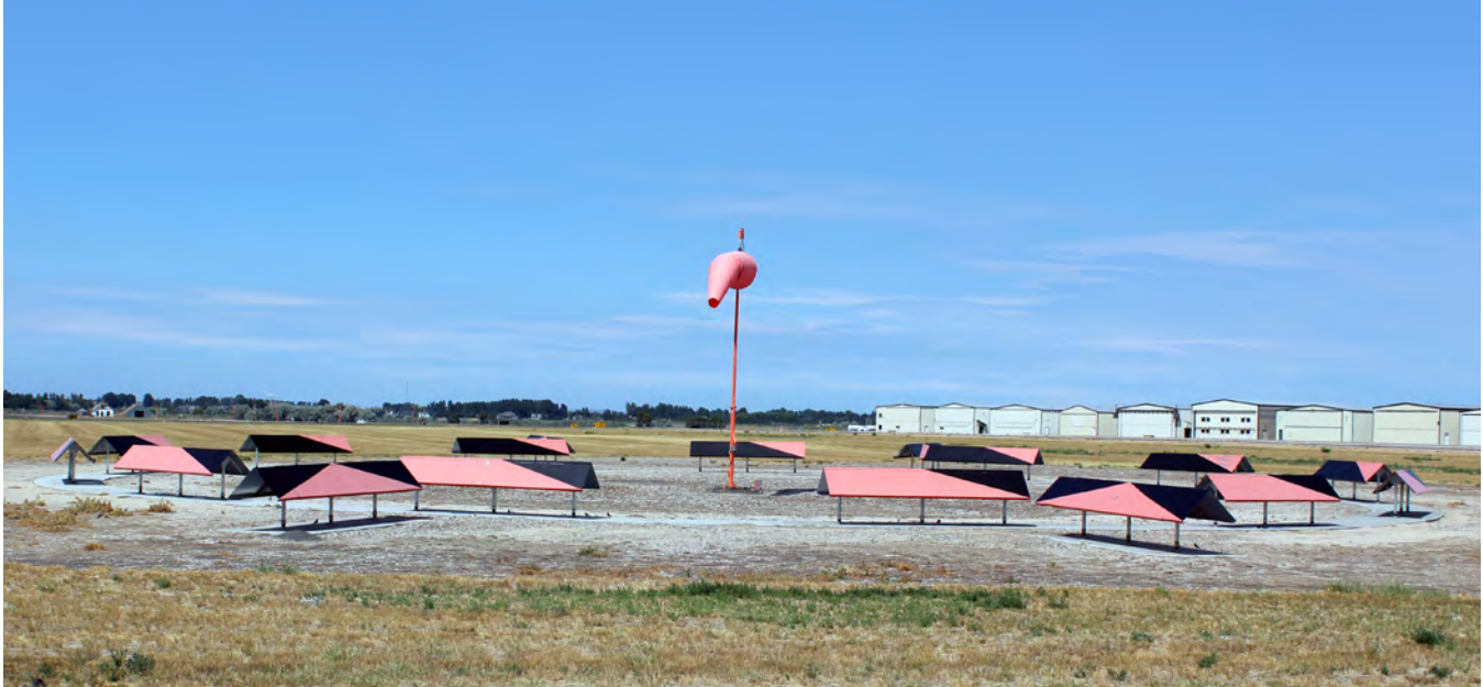
Figure 4.28: Segmented Circle and Lighted Wind Cone
