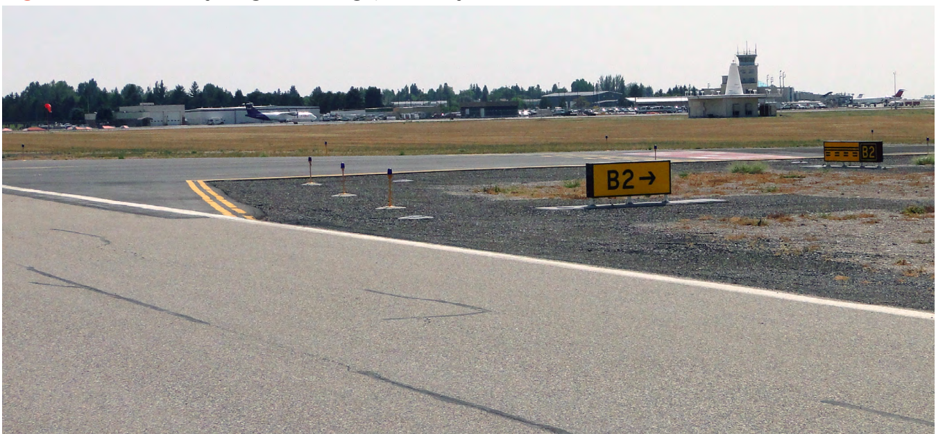
Figure 4.26: Runway Edge Markings, Runway 17/35
