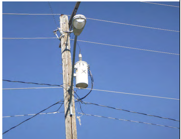
Pole mounted transformer adjacent to the subject property to the west.
