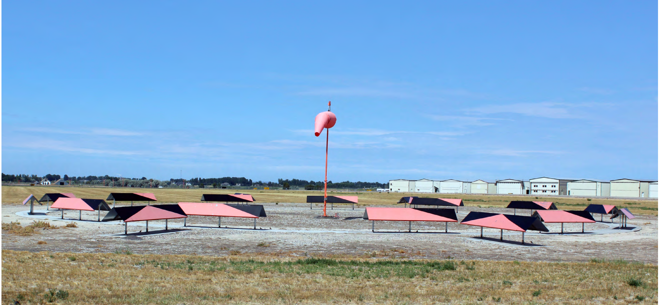
Figure 4.28: Segmented Circle and Lighted Wind Cone
