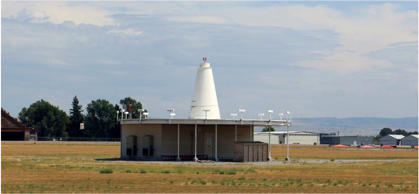
Figure 4.29: Very High Frequency Omnidirectional Range
