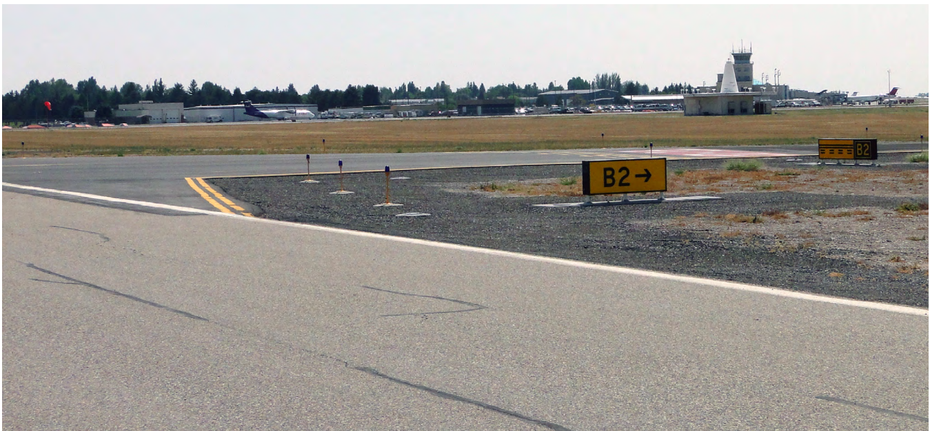
Figure 4.26: Runway Edge Markings, Runway 17/35
